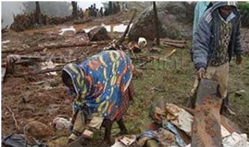
Figure 6. Picture of the area of Kapsokom where the landslide occurred. (Picture courtesy of standard newspaper dated 3 rd December, 2011)
